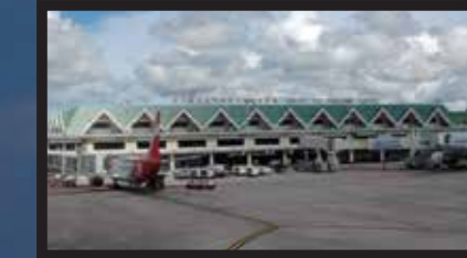
Phuket International Airport
